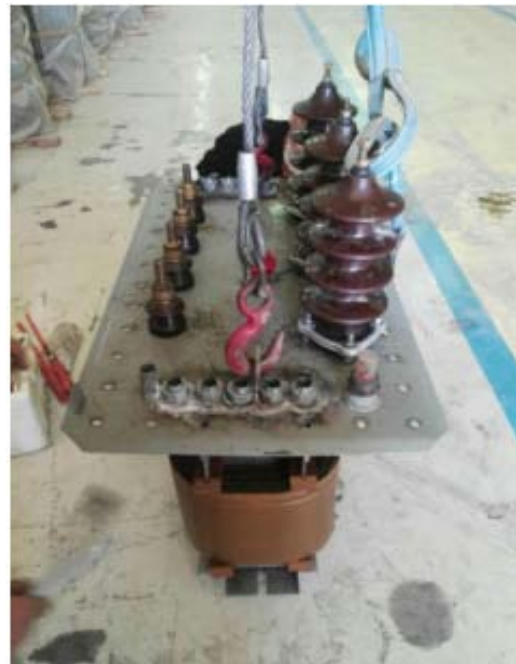
Fig. 4: Drill the top plate of the transformer
