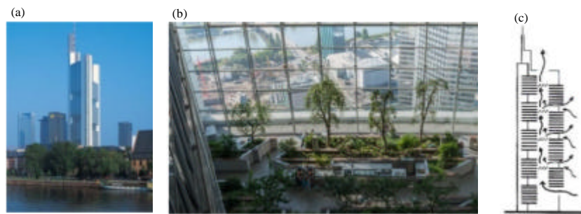
Fig. 3: a-c) Natural ventilation at the commercial bank regional management tower in Frankfurt, Germany
