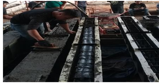
Fig. 5: Casting of specimen
