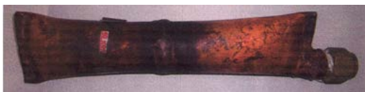
Fig. 6: Welded copper pipe (D = 40 mm) after hydrostatic test
