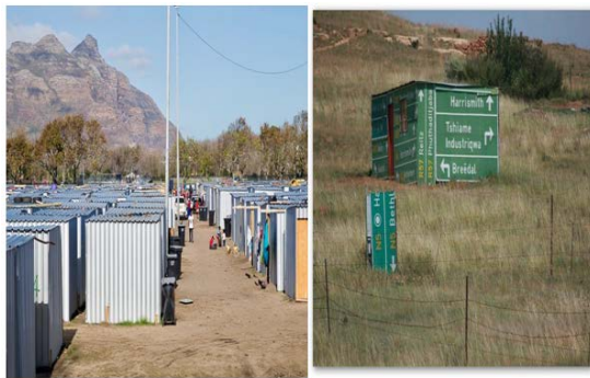
Fig. 5: Corrugated sheet and traffic signs used as materials for low-income household houses [25]
