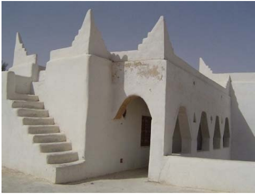
Fig. 9: A typical facade a traditional Libyan Arab house in Ghadames (Azzuz, 2000)
