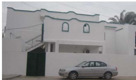
Fig. 5: A typical Arab house facade (min. external openings) illustrates symbolism and expressionism. Researcher's fieldwork in 2010
