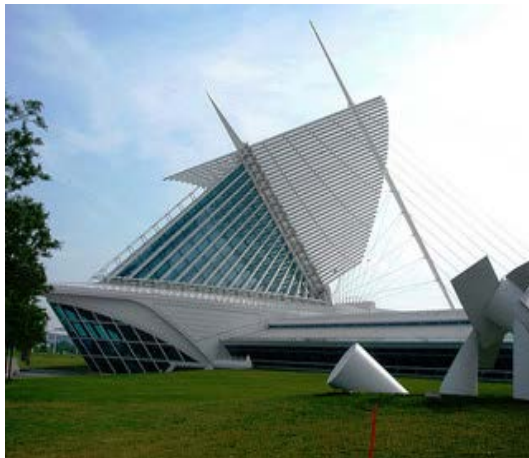
Fig. 8: Milwaukee art museum, Aantiago Calatrava in 2001 AD (www.greatbuildings.com)
