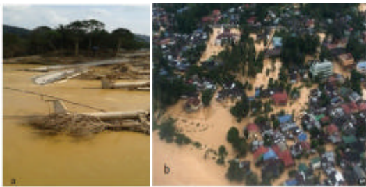
Fig. 1: Areas devastated by the floods: a) One of the bridges completely washed away by the floods and b) Parts of the towns completely submerged
