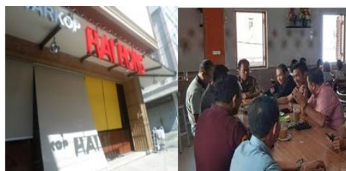
Fig. 7: Hai Hong coffee shop building after repairs and the atmosphere of visitors in a coffee shop; Personal Dokumentation, 2018
