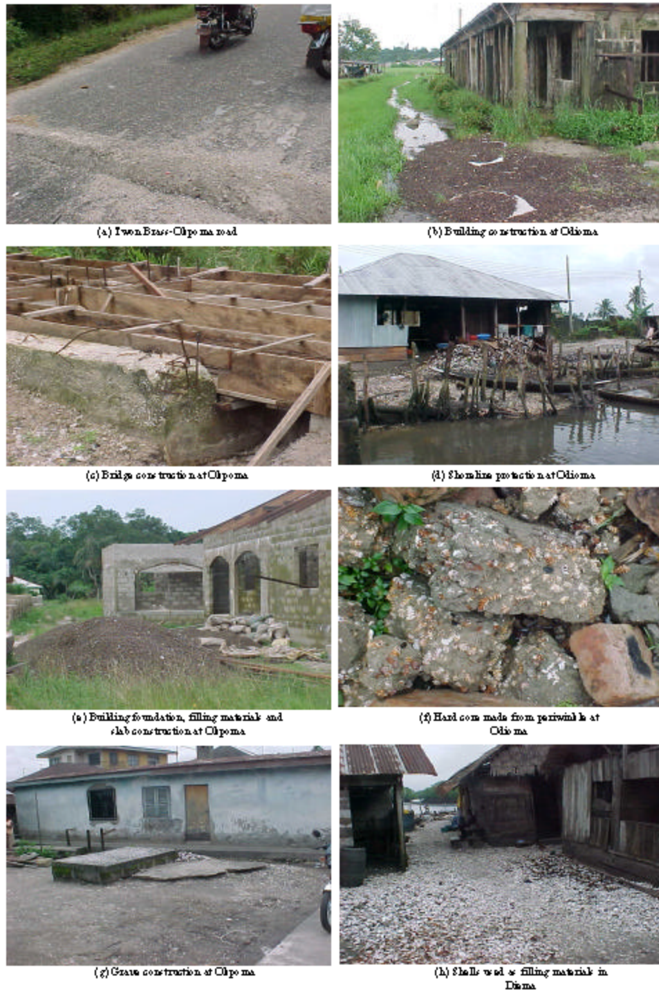
Fig. 2: The use of waste shells in civil construction works
