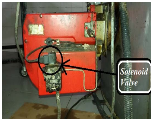
Fig. 3: Solenoid valve placement
