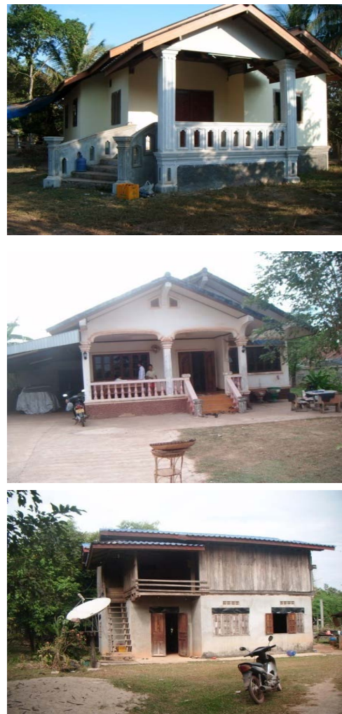
Fig. 6: Original house in Vientiane City
