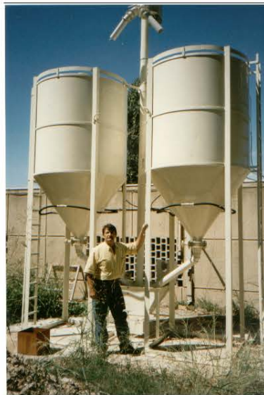
Fig. 1: Installation of the experimental two silos (3.5 tn each), with the following parts: (i) Screw conveyor (ii) Sensors for temperature and for relative humidity measurements (iii) inlet and outlet of gases (N 2 , O 2 )
