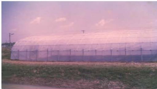
Fig. 1b: Outside view of the experimental greenhouse
