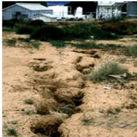
Fig. 3: Earth fissures will damage the structures
