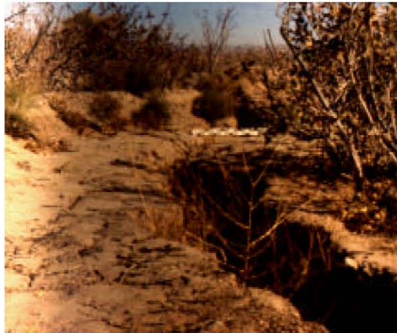
Fig. 4: Earth fissures among the pistachio trees in Sirjan land
