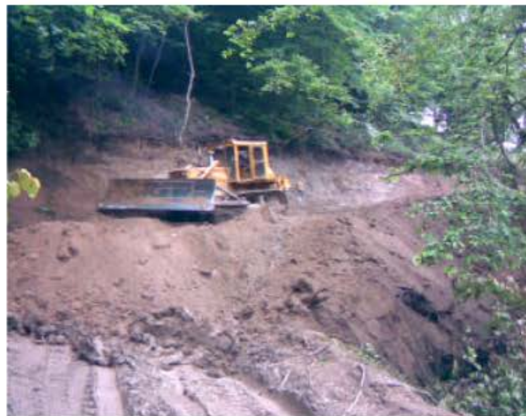
Fig. 3: Bulldozer earth working operation in study area
