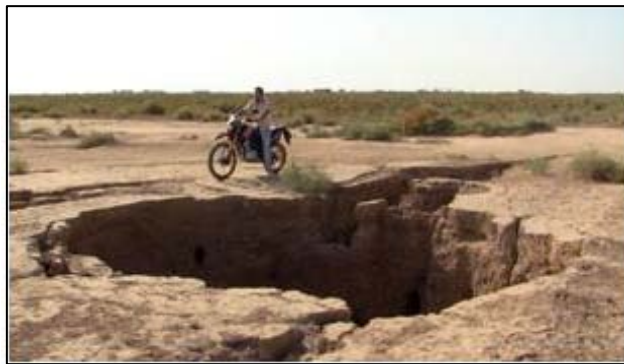
Fig. 2: Sinkhole in Sirjan well field land
