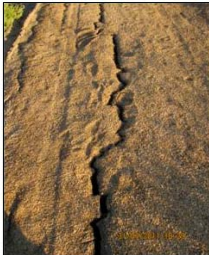
Fig. 3: Earth fissures in Sirjan (more than 1 km long)
