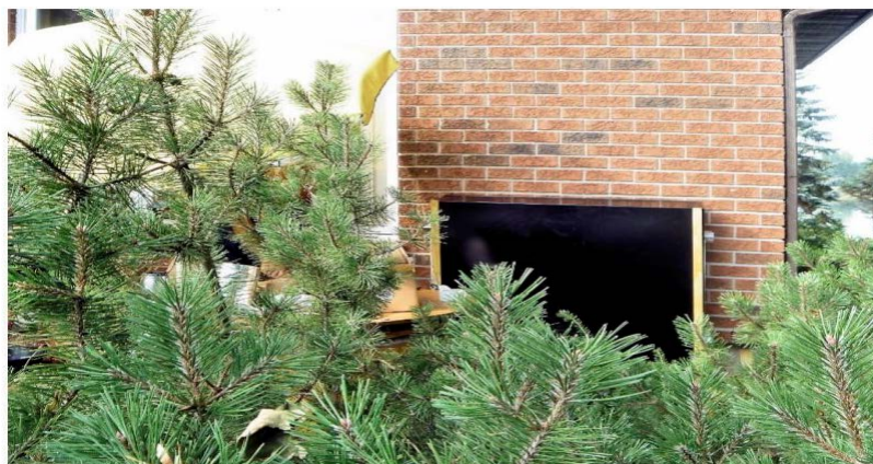
Fig. 4: Air-heat exchanger. The 50 kW air-heat exchanger transfers heat into the ground loop of the test-bed system
