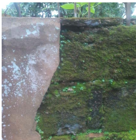
Fig. 5: Effect of surface roughness on the rate of biological growth
