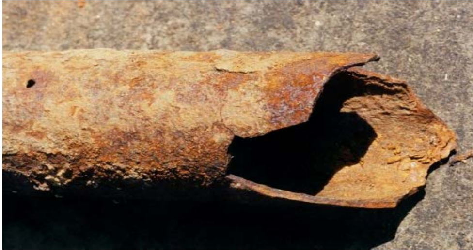
Fig. 2: Impact of corrosion on pipes used for pumping water
