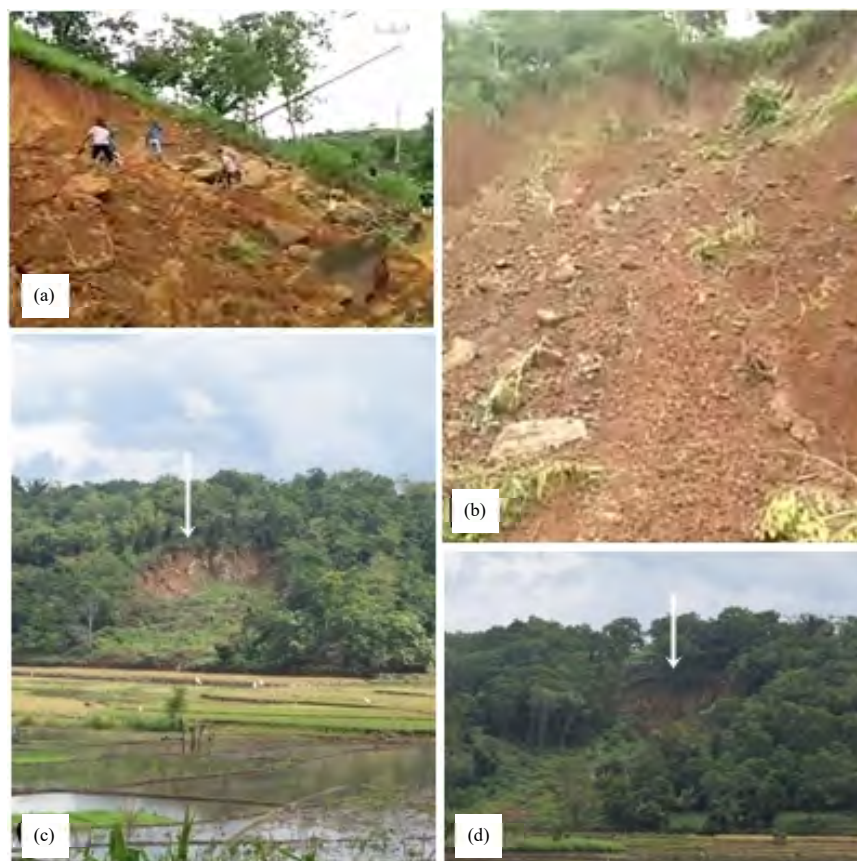
Fig. 9(a-d): (a) Appearance of several landslide events at sites 3 and 4 (b, c and d) On mixed plant land use in Rumbia District, Jeneponto Regency (the white arrow is landslides point)
