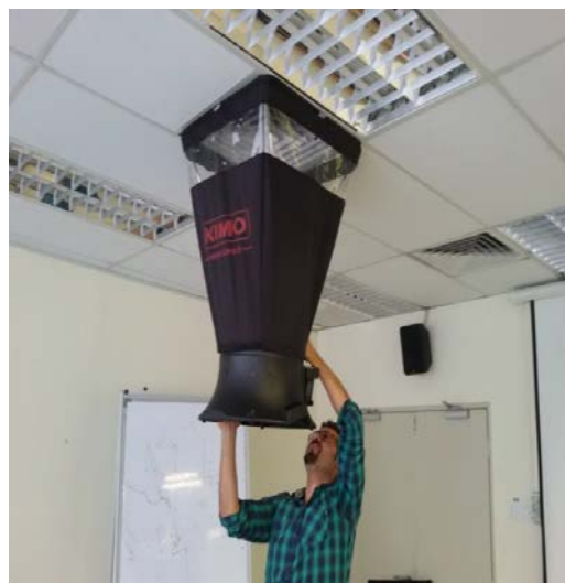
Fig. 5: Air flow rate measurement
