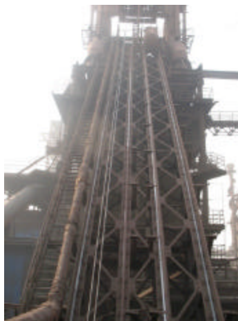
Fig. 1: Appearance of blast furnace skew bridge
