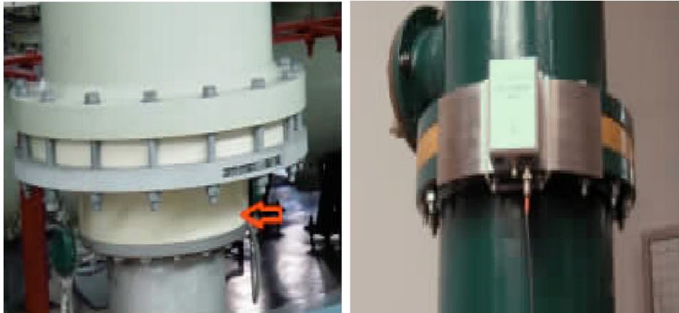
Fig. 3: Position of the UHF sensor
