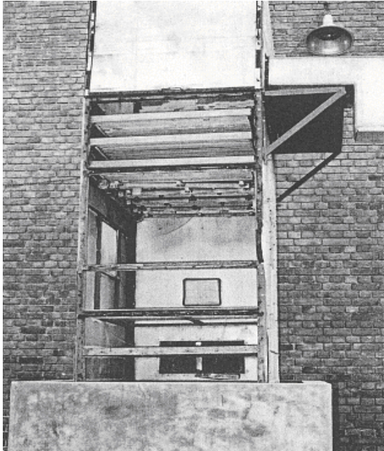
Fig. 3: Inside view of the test tower
