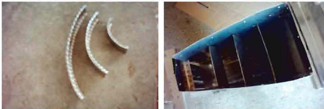
Fig. 6: Three separators installed in the air stream duct separating it into 4 sections
