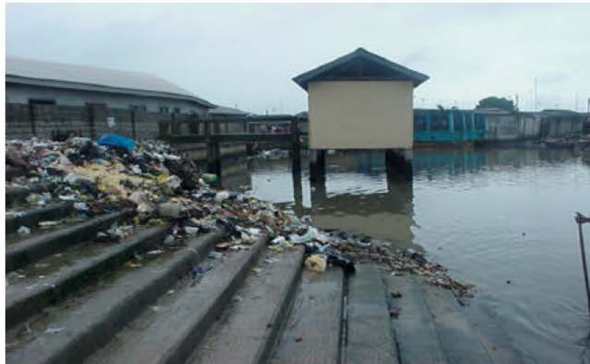
Fig. 1: A typical Overhung Toilet (Pier Latrine)
