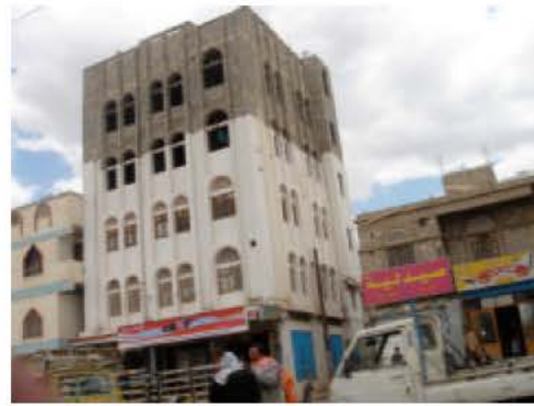
Fig. 2: The congested housing and buildings contiguity with each other, Sana'a
