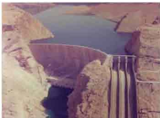
Fig. 1: Downstream view of Karoon-1 dam
