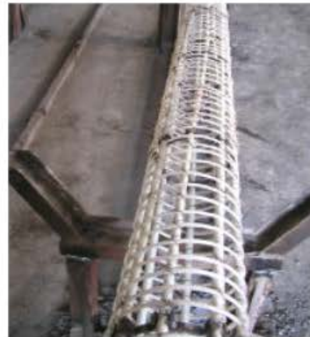
Fig. 1: The FRP reinforcement cage
