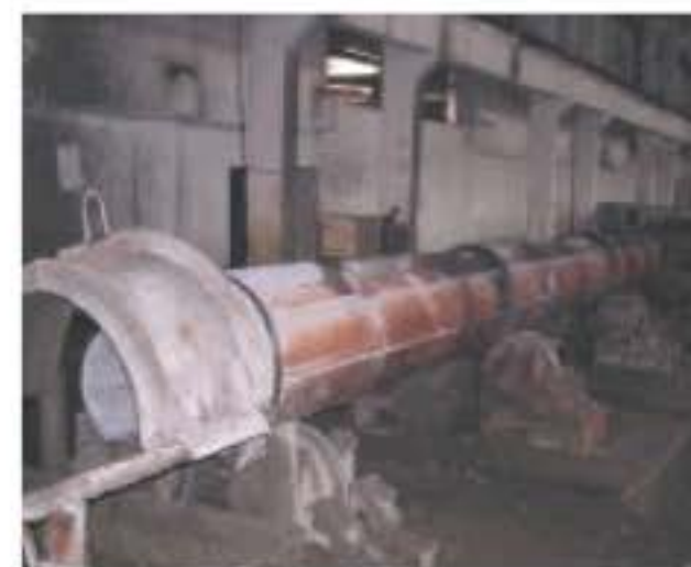
Fig. 3: The rotating wheels of the formwork
