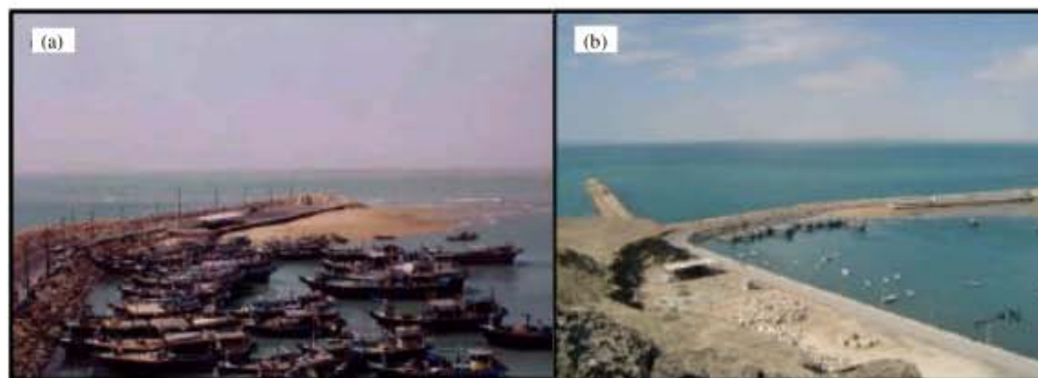
Fig. 2: (a) Sedimentation problem in the behind of South- North direction breakwater, (b) Two breakwaters layout of Pozm Bay
