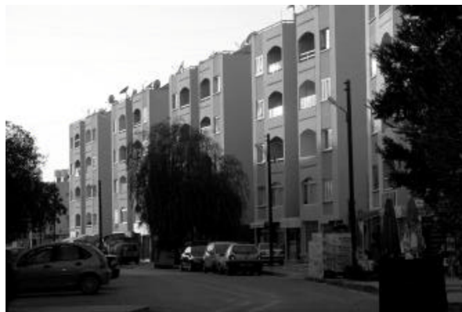
Fig. 1: The multi-storey social housing apartment development in Famagusta
