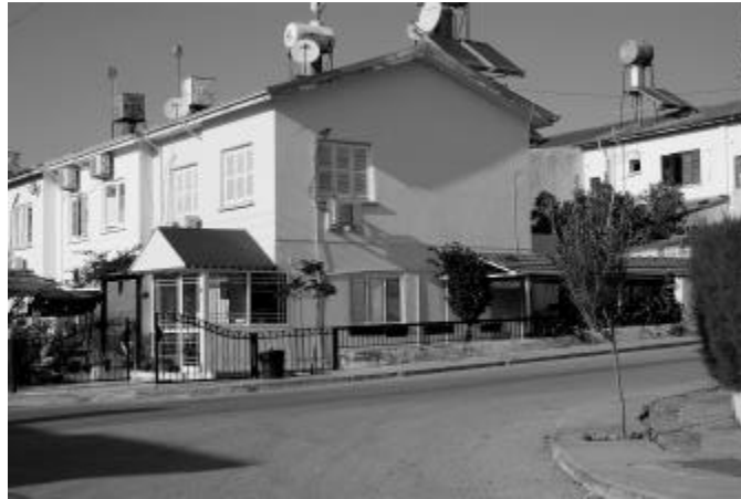
Fig. 2: A view of low-rise social housing in Sakarya district
