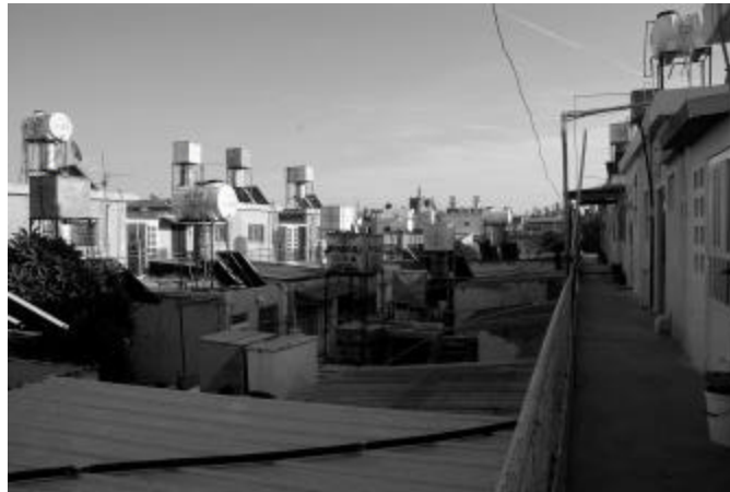
Fig. 10: Extensions to the backyards of the social housing in the walled city of Famagusta
