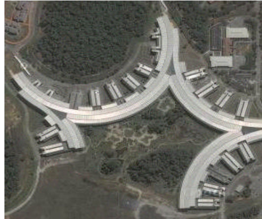
Fig. 1: Aerial view of the academic complex
