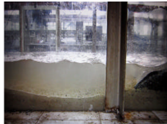
Fig. 12: Scouring pit in dam downstream
