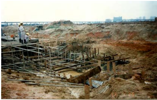
Fig. 5: The water and earth well up during construction
