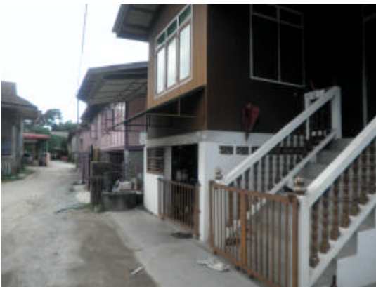
Fig. 6: Double storey house build by the people to faces the flood
