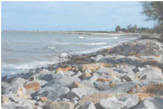
Fig. 3: Application of revetment to protect further erosion in vicinity of Sultan Mahmud Airport, Kuala Terengganu
