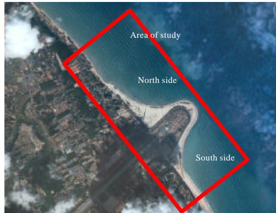
Fig. 6: North and south side of study area
