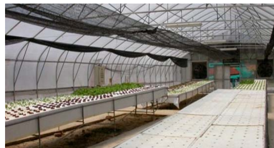
Fig. 2: Evaporative cooling, view of the fan end
