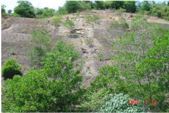
Fig. 3: Slope profile of the study area consists of 13 berms
