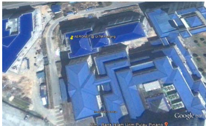
Fig. 2: AERONET installed on the roof of the academic block (BKBA) UiTM Penang. Map courtesy of Google Earth ®
