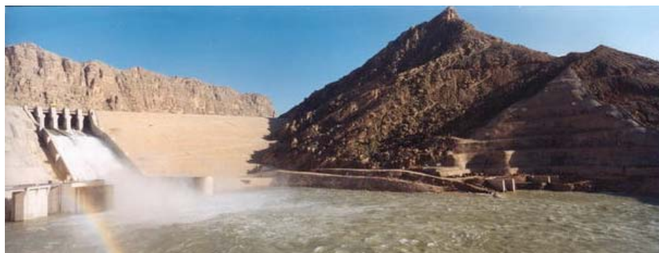
Fig. 2: Masjed Soleiman embankment dam; view from downstream
