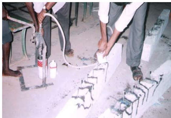
Fig. 2: Injection of epoxy resin on beams
