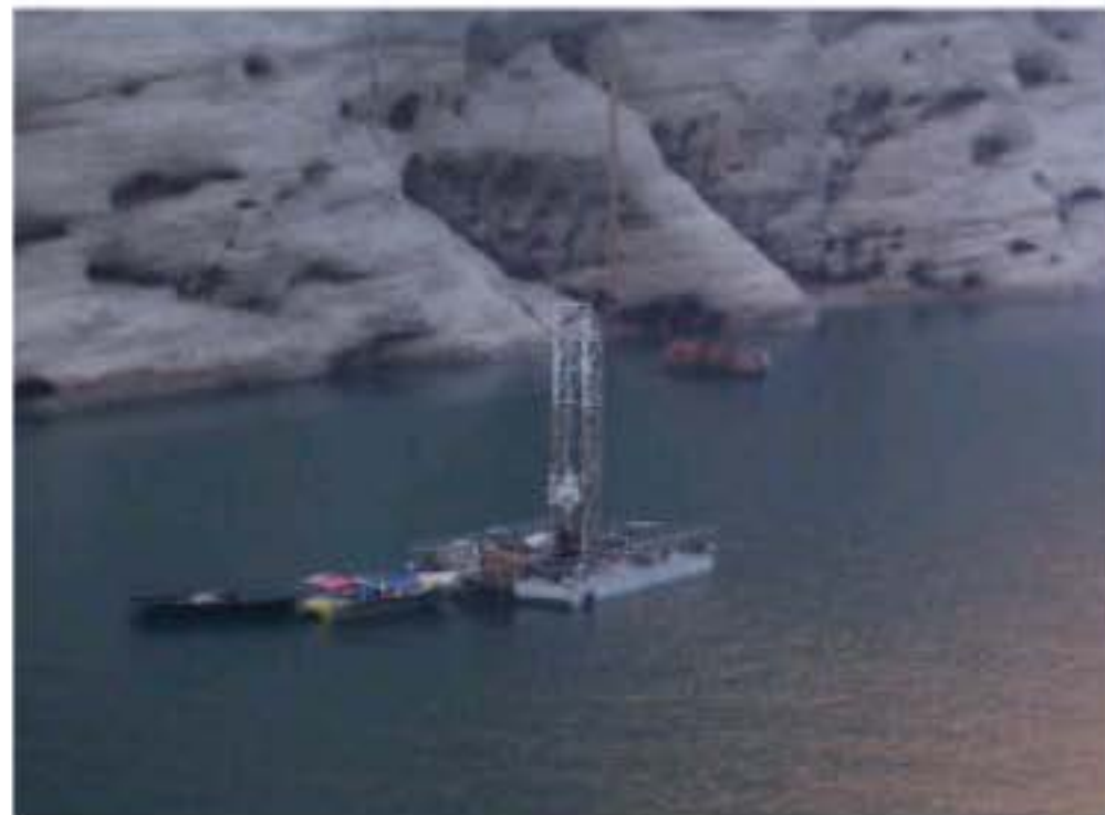
Fig. 3: Photo of barge and digger located near Dez Hydropower intakes
