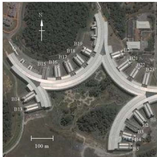
Fig. 1: Aerial view of the academic complex
