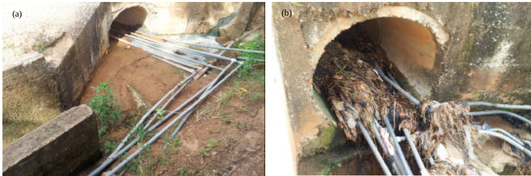
Fig. 1(a-b): Water distribution systems among drianage system, (a) Solid waste and (b) Connecting drinking water from the main overhead distribution tank to domestics outlets at Appeadu in Kumasi, Ghana
