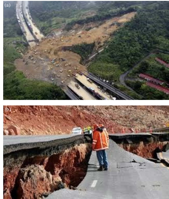
Fig.1(a-b): Landslide along Calabar-Itu highway in Akwa Ibom state, Nigeria
